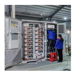
The project is expected to be made up of 608 Z3.4 Cube energy storage units manufactured by Eos Energy, utilising its zinc hybrid cathode aqueous electrolyte battery technology.
