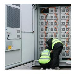
To address the safety issues associated with lithium-ion energy storage, NFPA 855 and several other fire codes require any BESS the size of a small ISO container or larger to be provided ...
