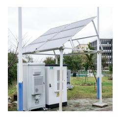
The mobile solar container system includes solar panels, storage batteries, inverter, mounting brackets, and accessories. Solar panels collect energy from the sun and store it in the battery ...
