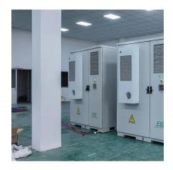
The EESS is composed of battery, converter and control system. In order to meet the demand for large capacity, energy storage power stations use a large number of single batteries in series ...
